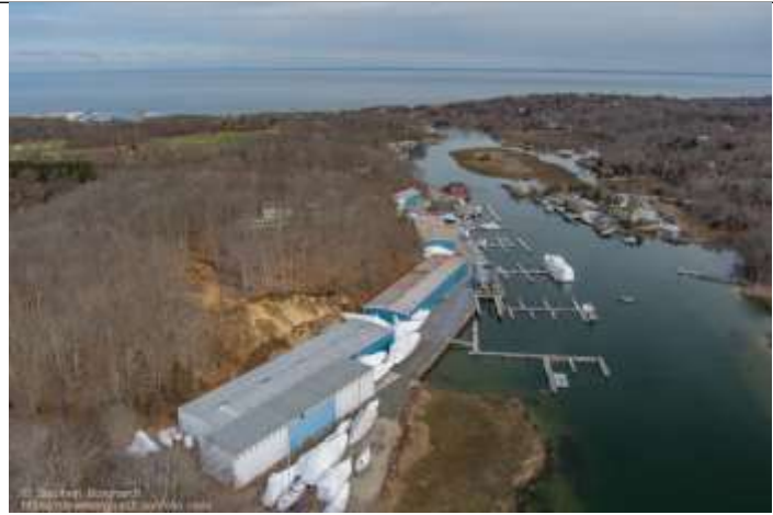
Mattituck Inlet Overhead photo of Strong's Marina Development site – photo by Stephen Borghardt
