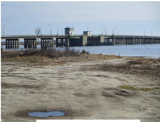
The current bridge
