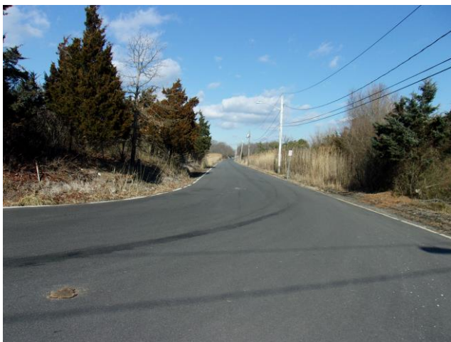
Newly paved road
