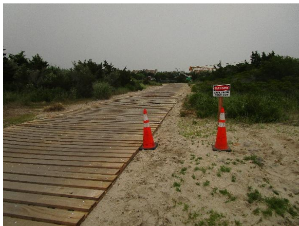
Construction begins on new bridge
