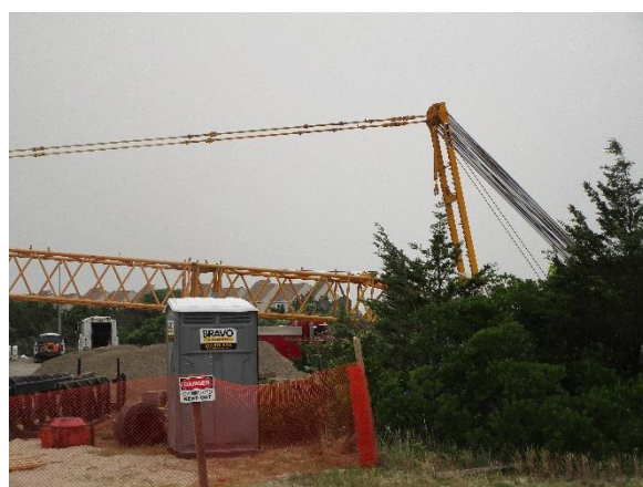
The new bridge is scheduled to be opened on 2029
